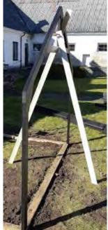
Attach the roof beam to the front and back wall (metal brackets are already attached to the roof beam). Fasten with screws 5x40 (4pcs)
