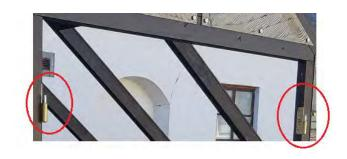
NB! OPENING A DOOR WITHOUT THE DOOR STOPS INVOLVES DANGER TO BREAK THE SIDE GLASS (the door handle goes to the side glass. It is definitely necessary to limit the turning area of the door!)
